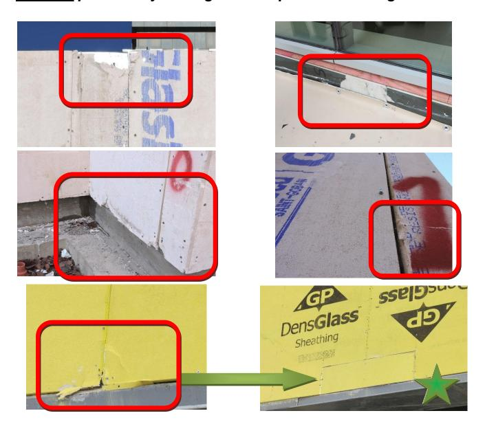
When the paper face is torn off, the roof adhesive or the air/vapor barrier will get sucked into the gypsum and not properly adhere.
